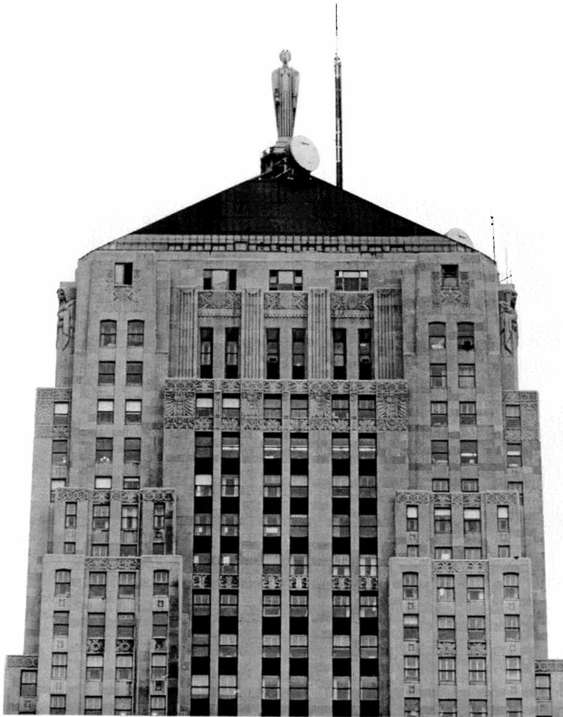
The top of the Chicago Board of Trade Building, with low-relief Art Deco-style sculpture defining the building's setbacks. Atop the low pyramidal roof rises Ceres , designed by artist John Storrs in an abstract style reflecting the influence of early 20th-century French modernism.
